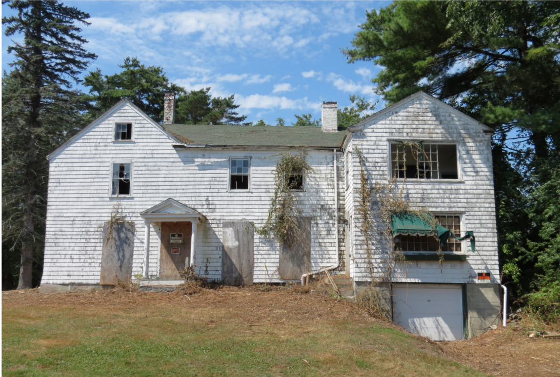
Photo 21: View of east elevation.
