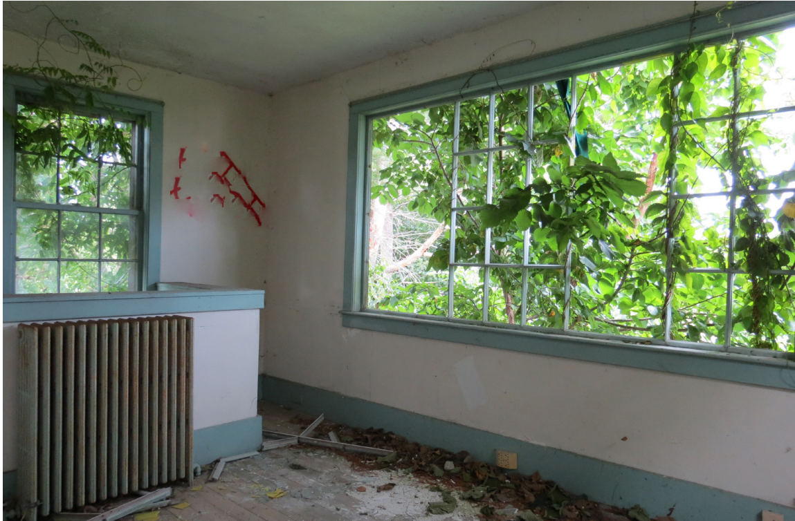
Photo 49: View in second floor sun porch.
