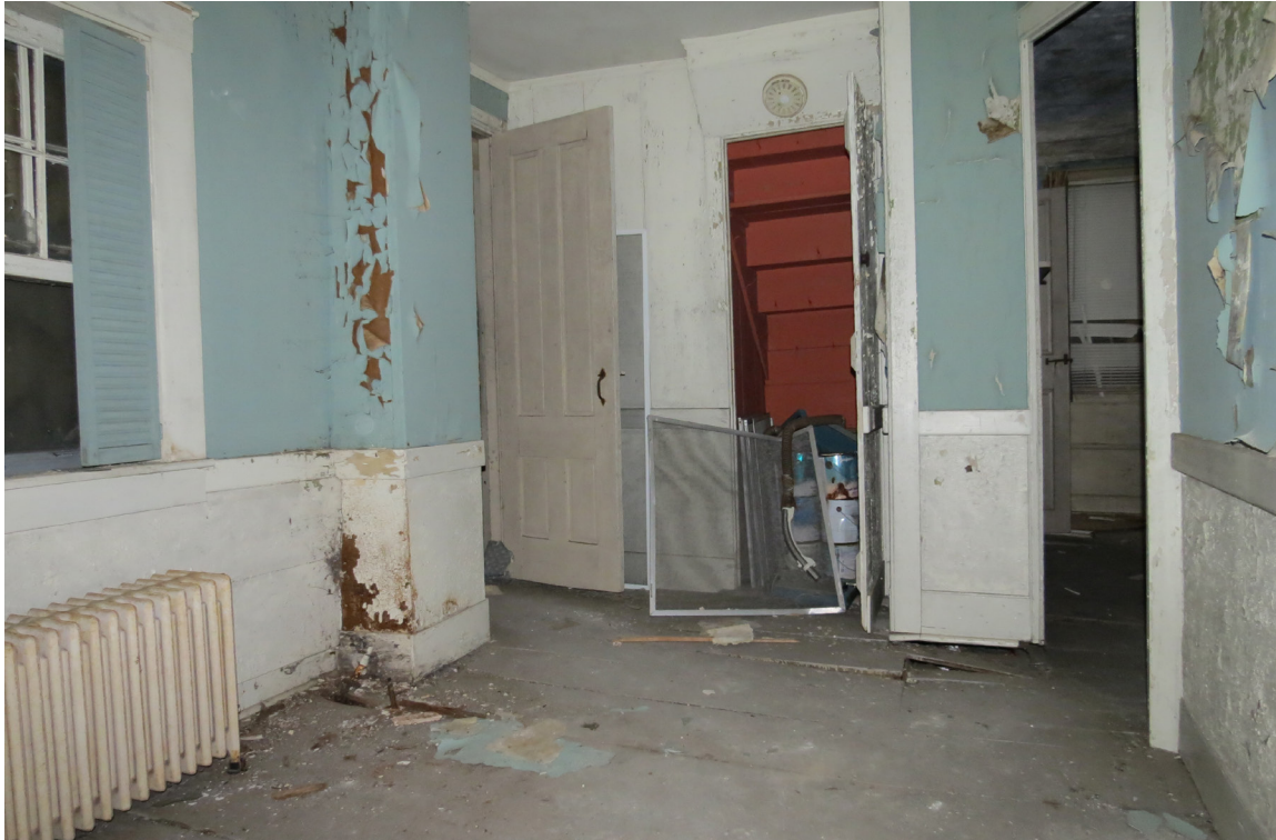
Photo 31: View in back room.
