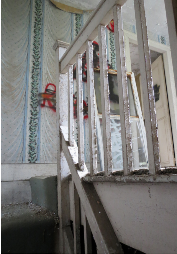
Photo 43: Front stair detail.
