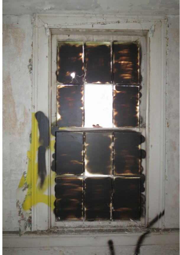
Photo 14: Federal style window trim and chair rail sill.
