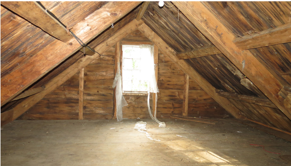
Photo 52: View in attic. Not keyed.
