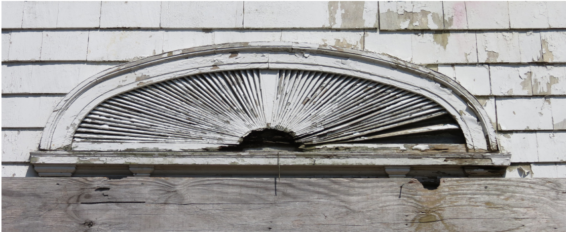
Photo 1: Front door surround including elliptical louvered fan.
