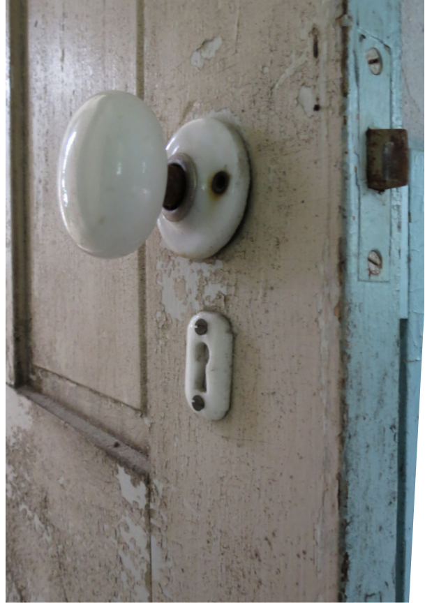
Photo 51: Detail of Victorian era door hardware in second story of ell. Not keyed.
