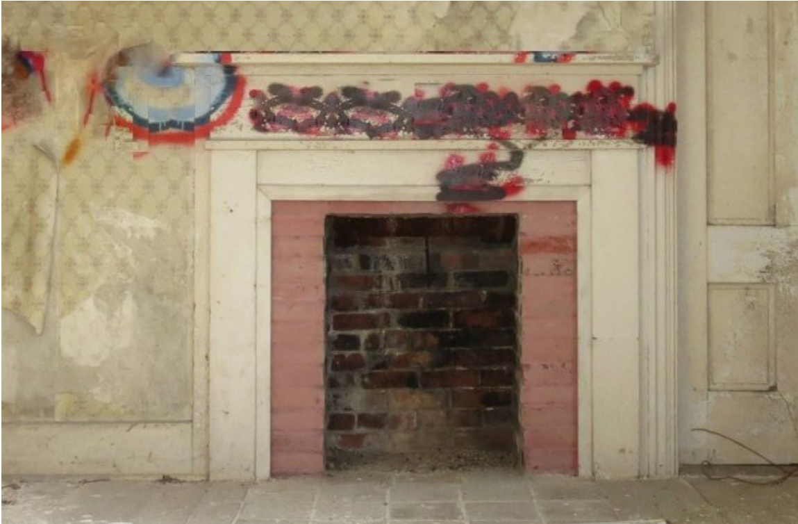
Photo 12: Greek Revival Mantel in bedroom.
