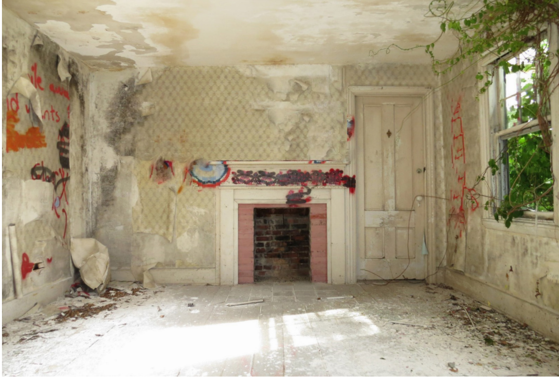
Photo 46: Room view in ell bedroom.
