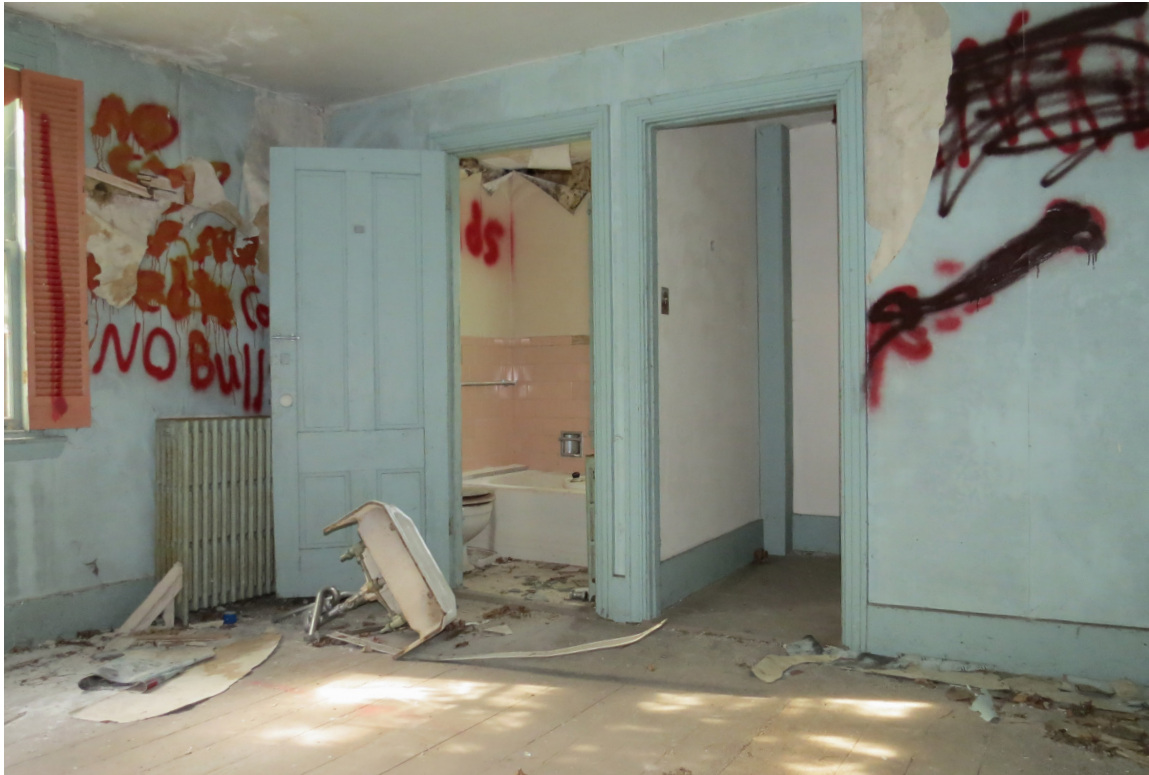
Photo 48: View in second floor back room.
