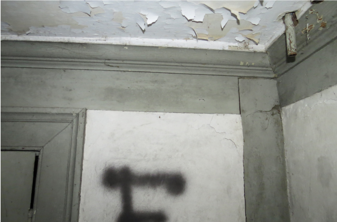
Photo 29: Federal style trim details in living room.
