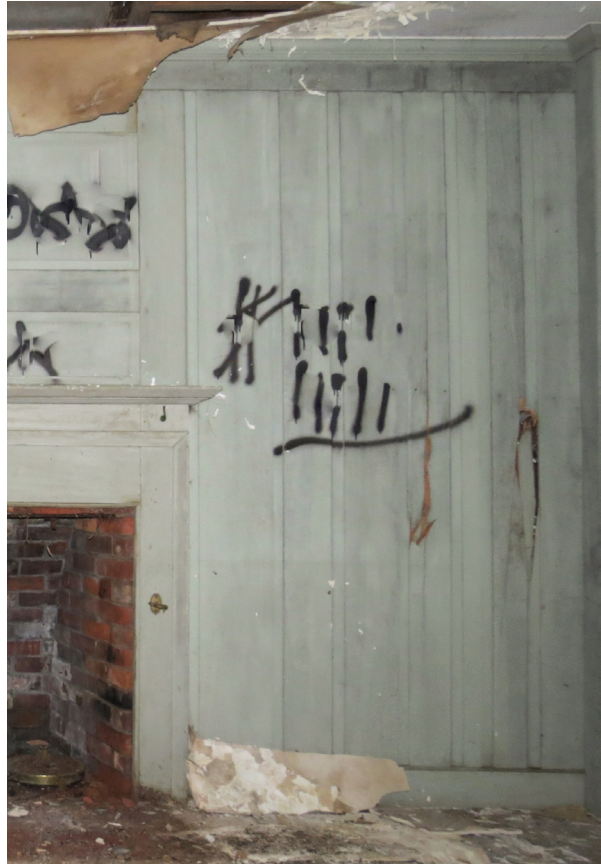
Photo 9: Vertical wide board paneling.
