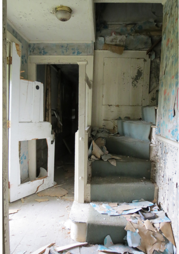
Photo 37: View of side hall and stair.
