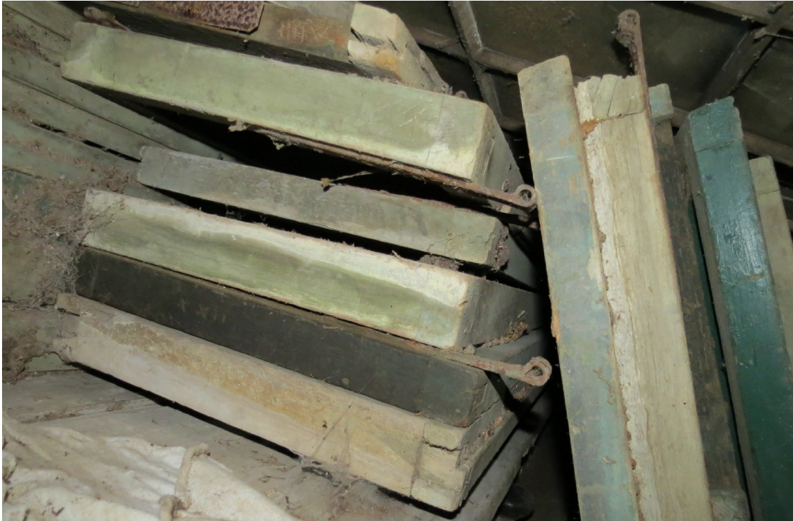
Photo 2: Early louvered shutters with hand-forged hinges (stored in garage). Not keyed.
