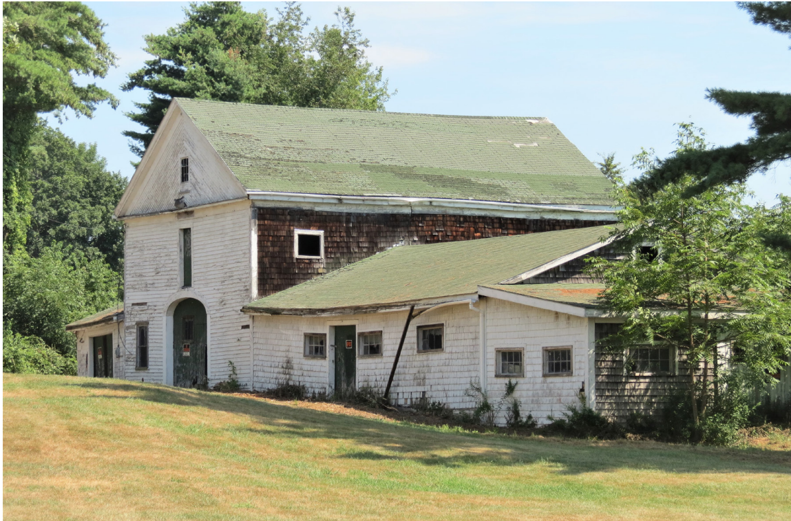
Photo 54: The two-story 19th century portion of the barn retains its historic clapboard siding and trim on the facade.
