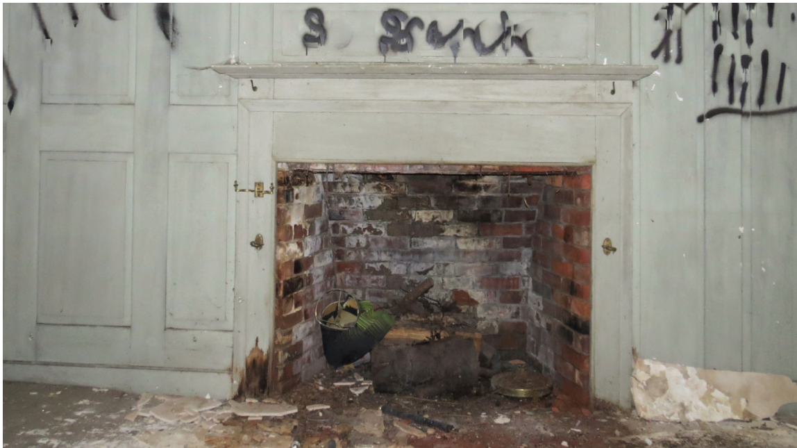
Photo 10: Federal Style mantel in living room. This chimney was moved at some point and the mantel and paneling relocated. Note raised panels on one side of the mantel and vertical board on the other.
