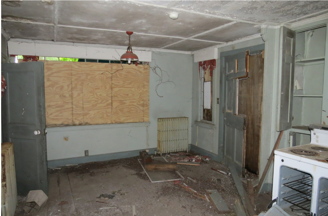
Photo 35: View in kitchen.
