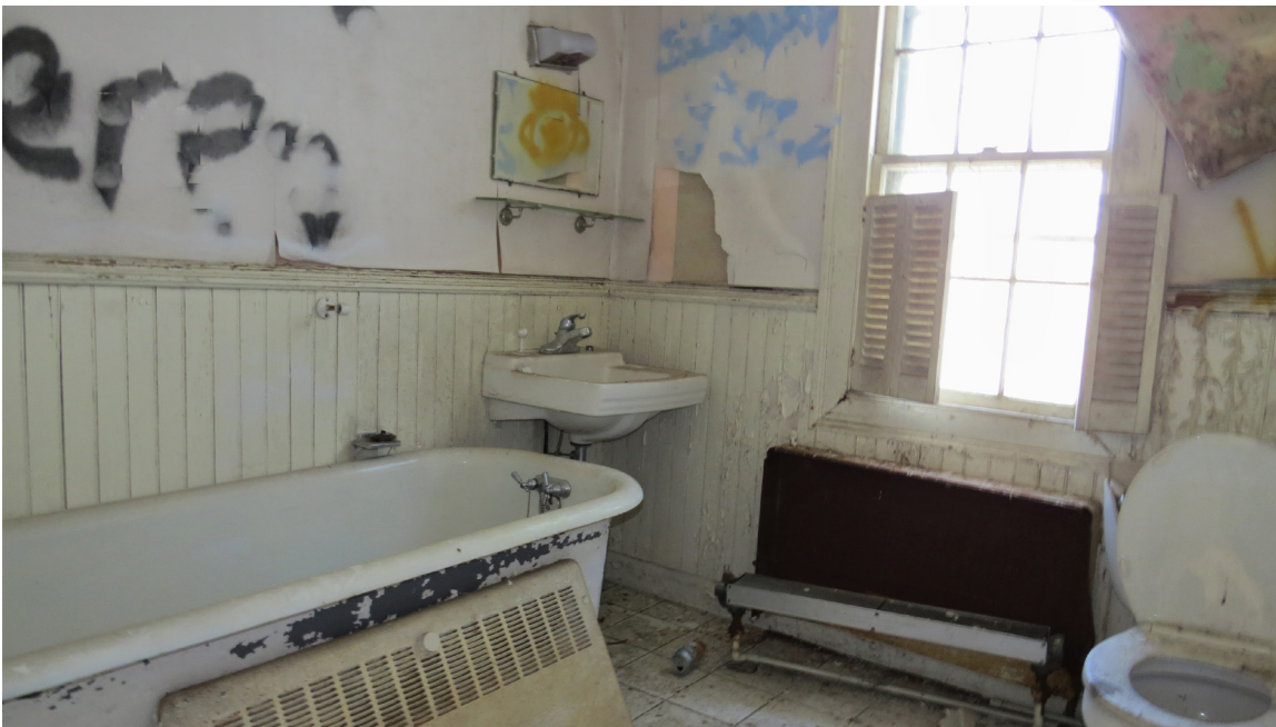
Photo 45: Bathroom off front stair.
