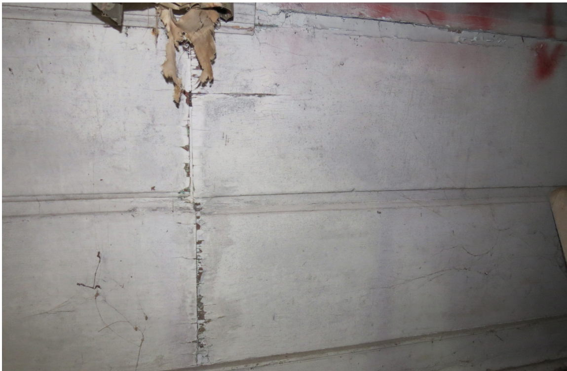
Photo 7: Horizontal wide board wainscoting.
