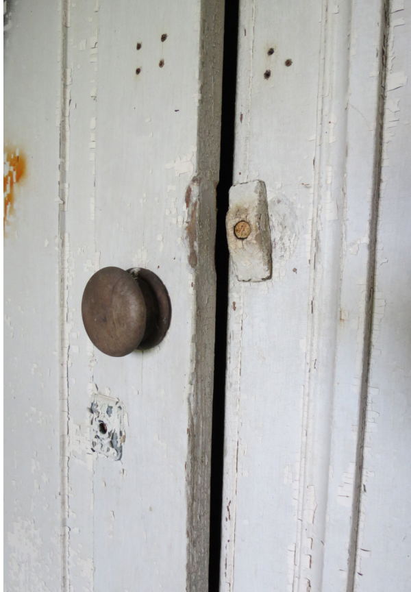
Photo 13: Federal style door trim and hardware.
