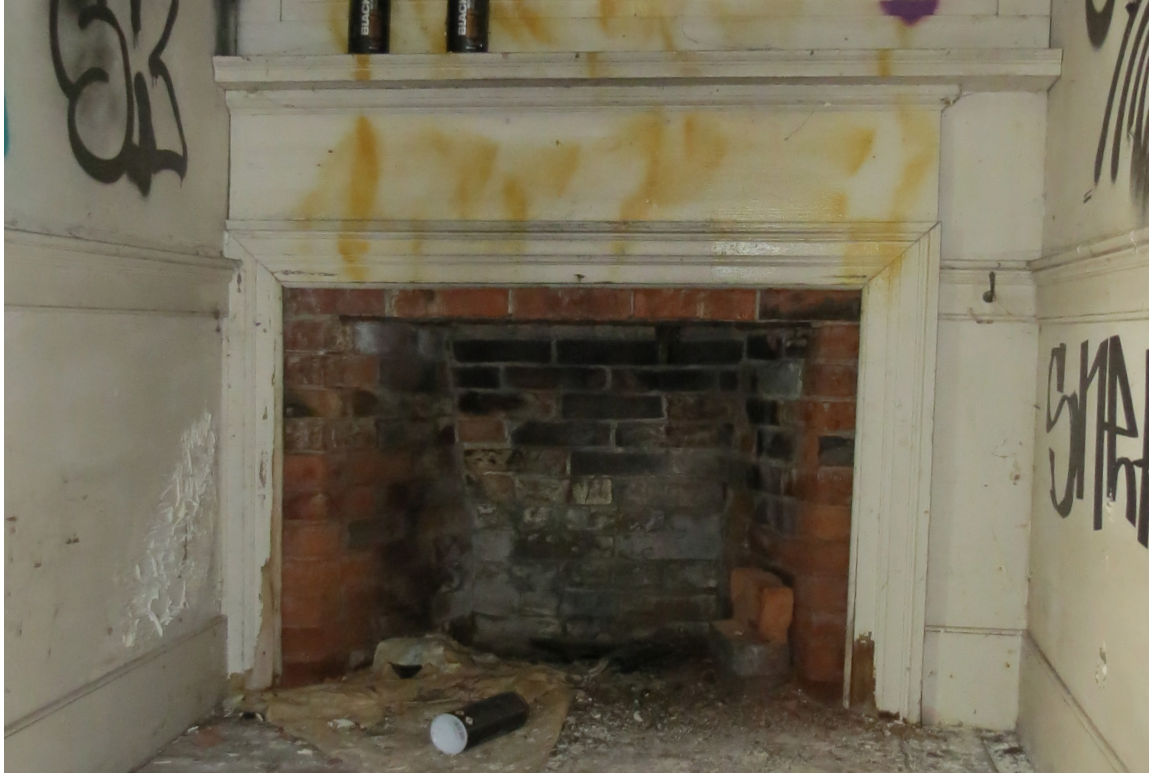
Photo 11: Federal style mantel in bedroom
