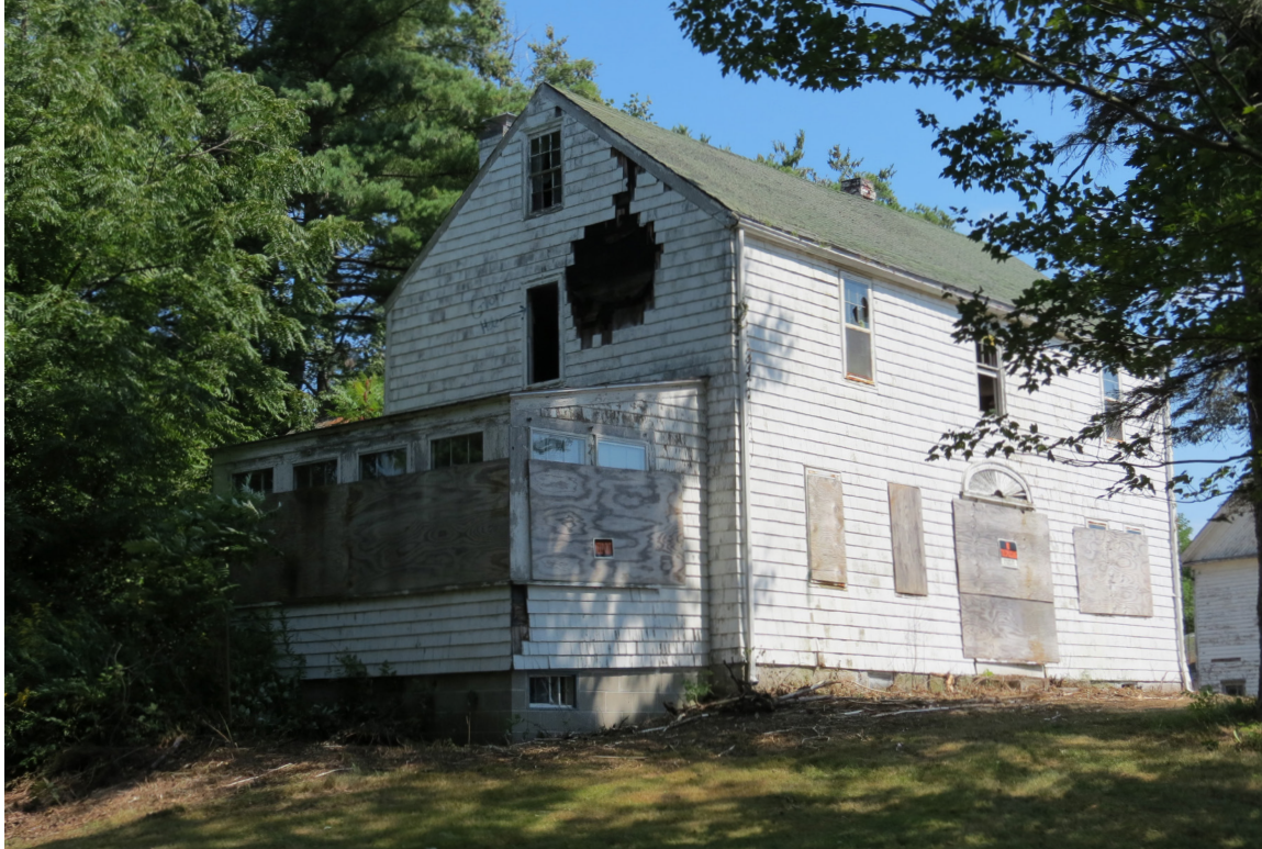
Photo 19: View of west elevation and facade.
