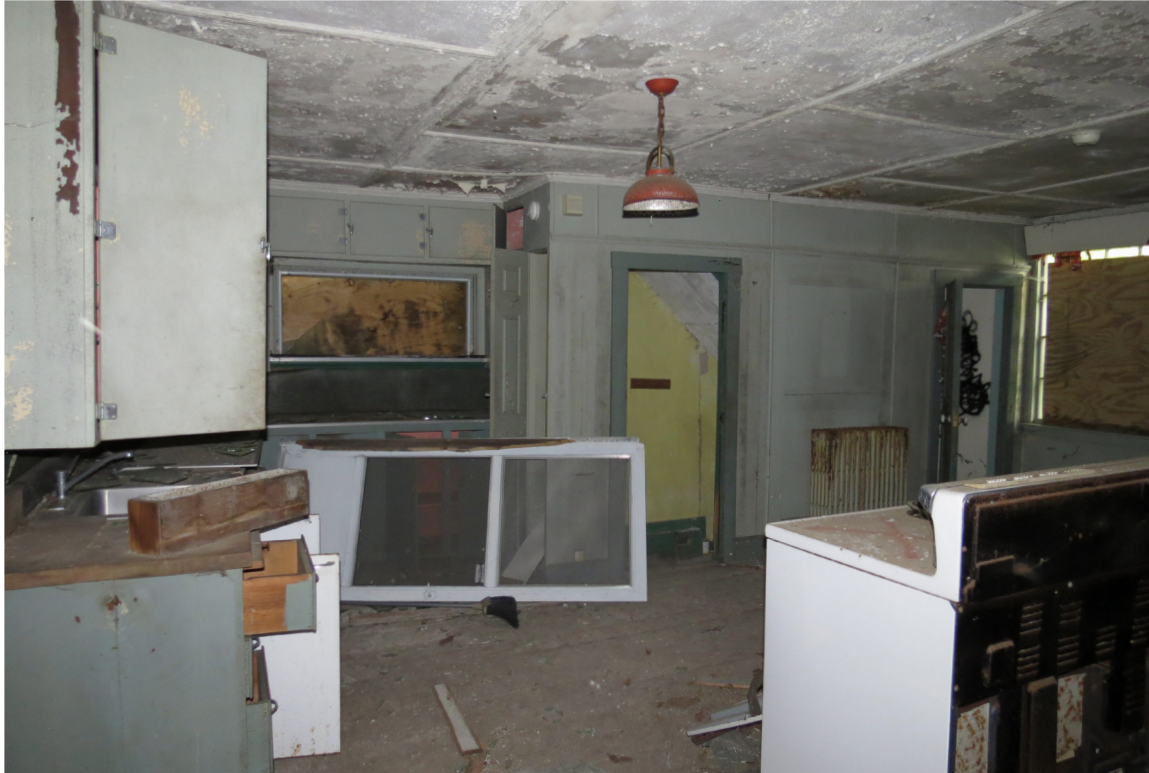
Photo 34: View in kitchen
