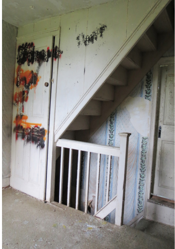
Photo 44: Second floor front hall.
