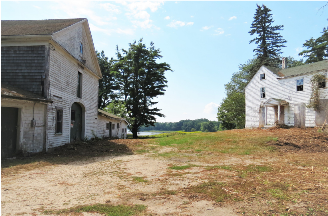
Photo 53: View showing the relationship of the barn and house.
