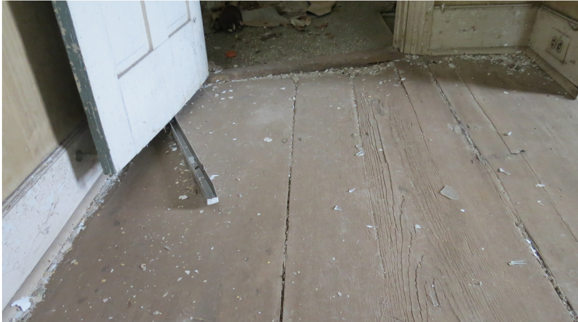
Photo 6: Wide board pine floors (some boards exceed 24" width).
